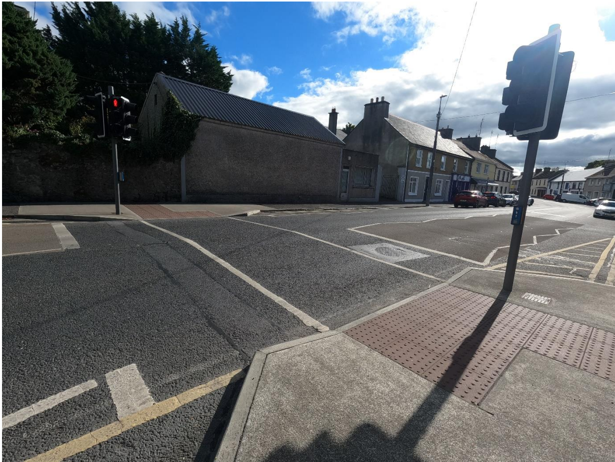
Figure 3-22: Church Road Signalised Crossing
