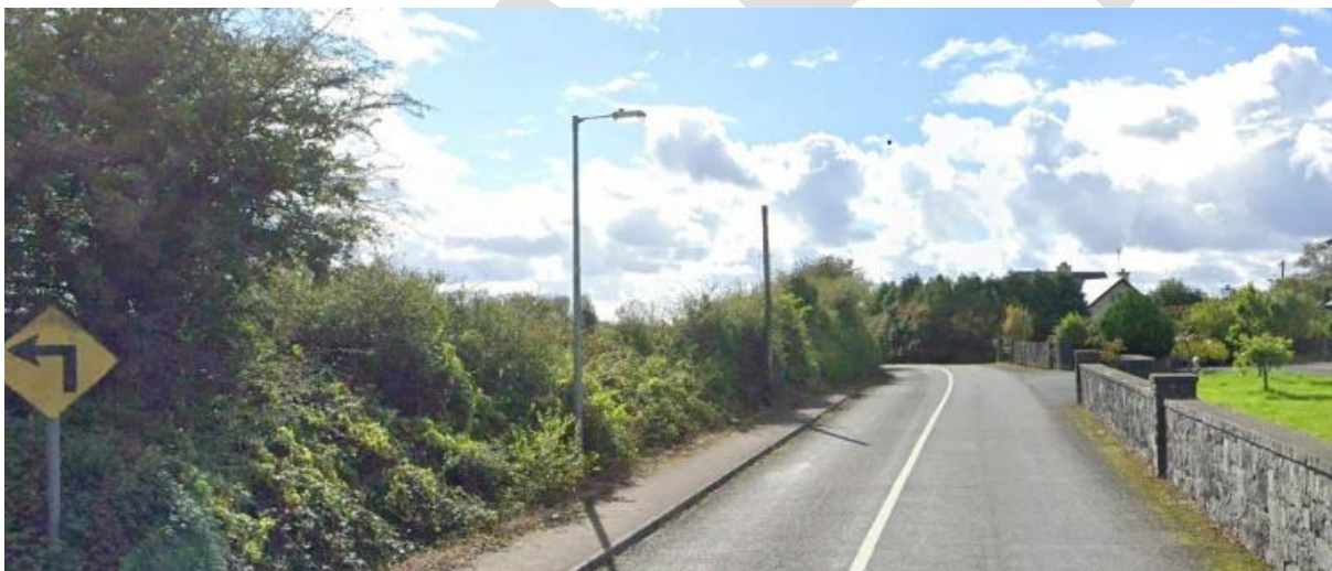
Figure 6-8: Missing footway at blind bend on Glenbrack Road
