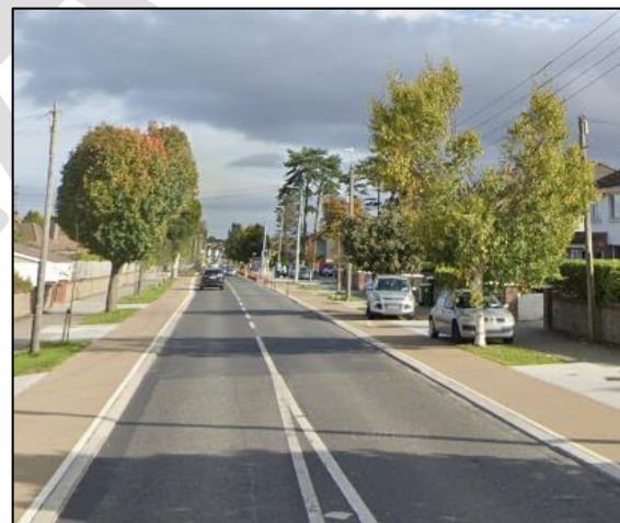
Figure 5-2: Example of a Segregated Cycle Track
