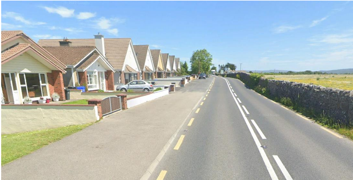
Figure 6-9: New housing and wide footway on Loughrea Road looking towards Loughrea
