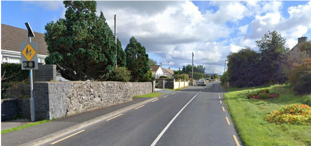
Figure 6-7: Missing footway along R460 looking towards Tubber Road
